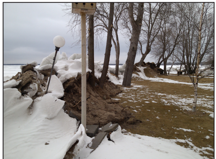
Ice damage is concentrated on the south shore of Otter Tail Lake rather than the north shore.
